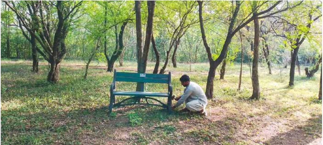
Installation of benches and dustbins at Trails 3 and 5 in Islamabad during 2025 to improve visitor convenience and promote cleanliness
